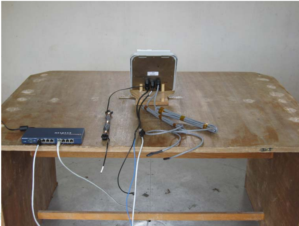
Test set up (POE switch)
