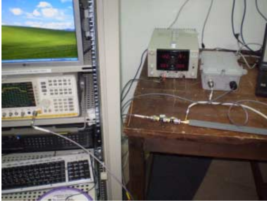
Photograph No.2 Occupied bandwidth and spurious emissions measurements at RF antenna connector test setup
