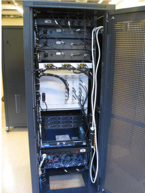
Figure 6: ABR757 Rear view picture
