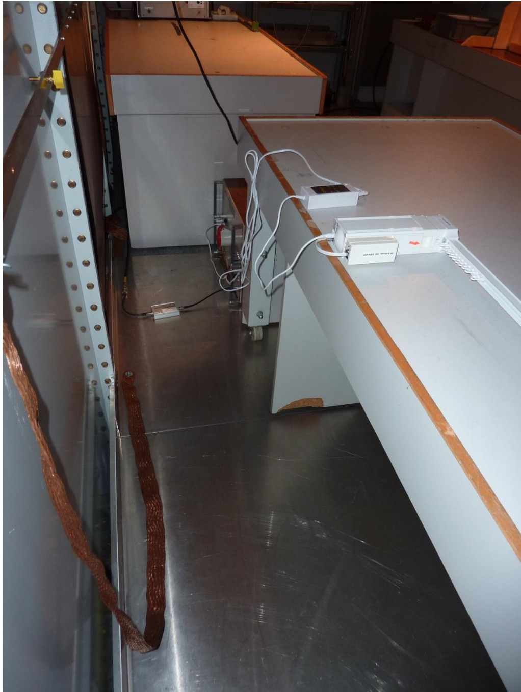
170813_9.JPG: Transceiver PV, shielded chamber
