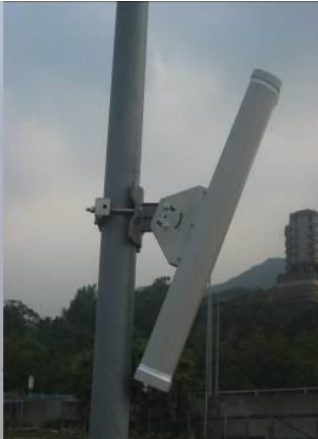
Figure 18. Adjust A8n 2.4GHz Antenna tilting
