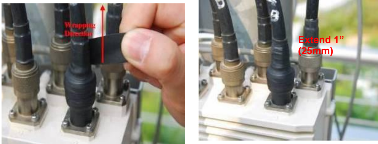
Figure 29. Wrapping direction and extends the wrap 1" above the connector clamping
