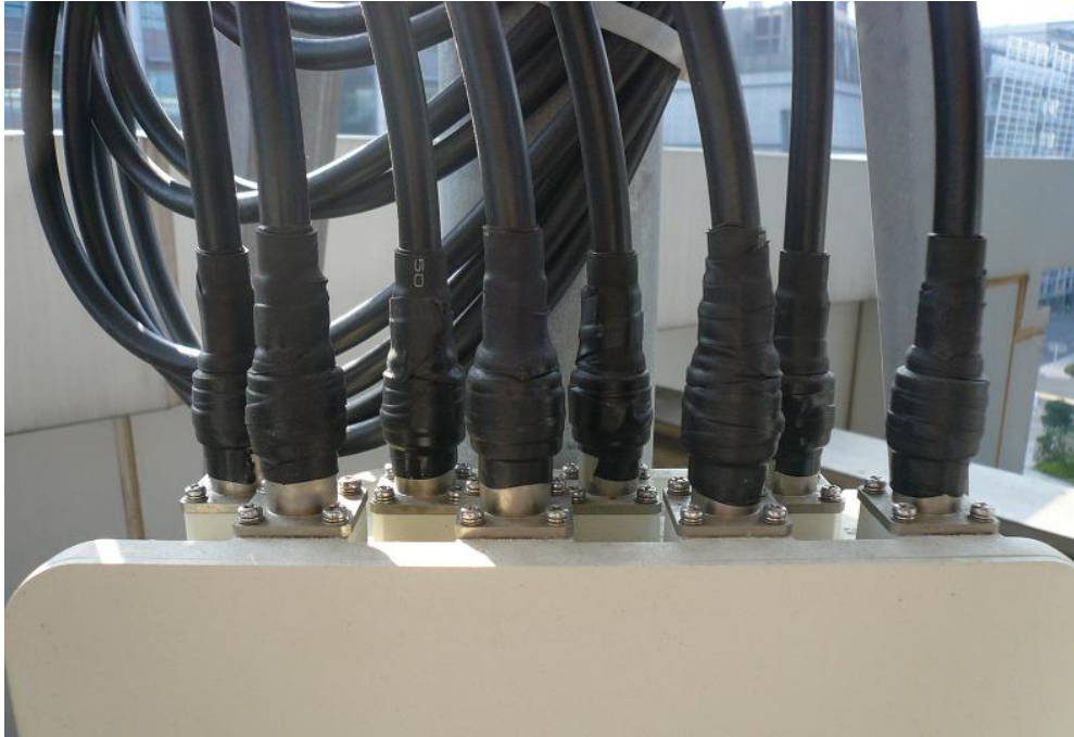
Figure 27. Wrap the Butyl Rubber Strip
