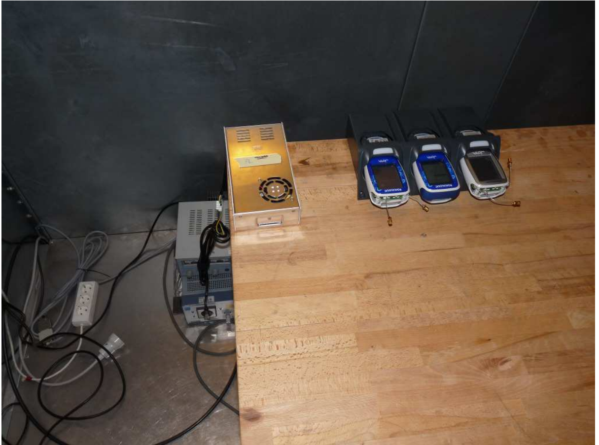
Test Setup (conducted measurement) Setup with AC/DC converter
