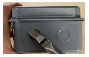
For ¾" knockout first use screwdriver to punchout ½" knockout then use pliers to remove outer ring.
