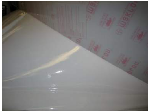
Figure 63: Scratch Guard Film Being Removed
