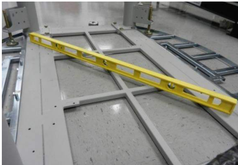
Figure 44: Cross-Level Check
