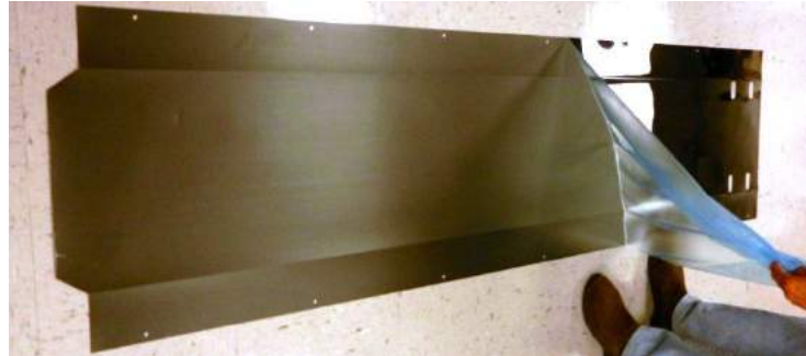
Figure 58: Cosmetic Mast Wrap Protective Film Being Removed
