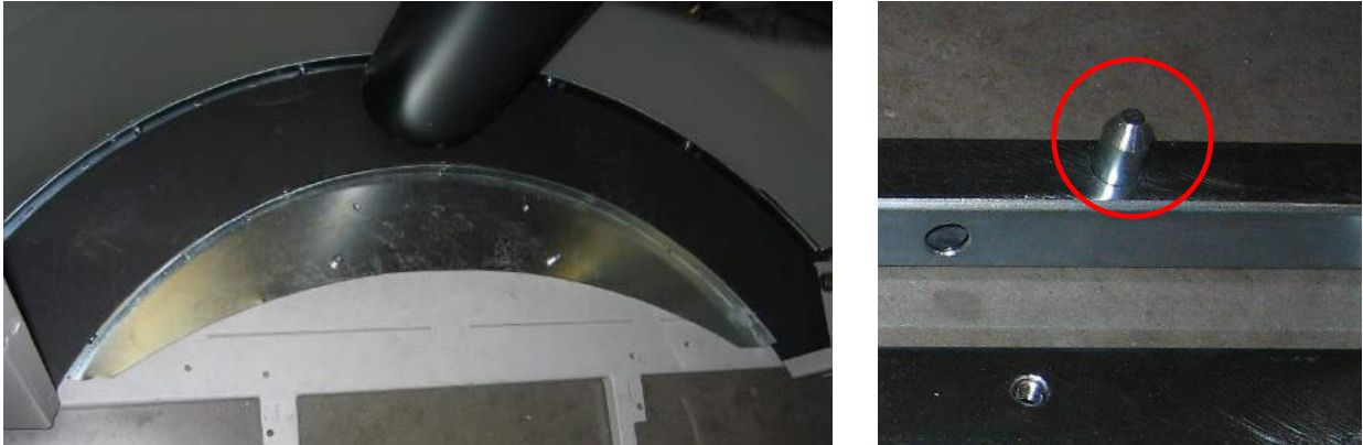
Figure 82: Inner Radome Base Flange Support Bracket and Guide Pin
