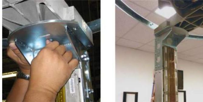
Figure 54: Antenna Mast Being Attached to Swing Arm
