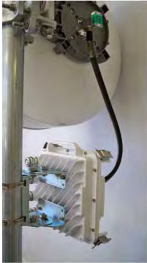
Figure 13 Remote-mount pole mounting mechanics, horizontal orientation
