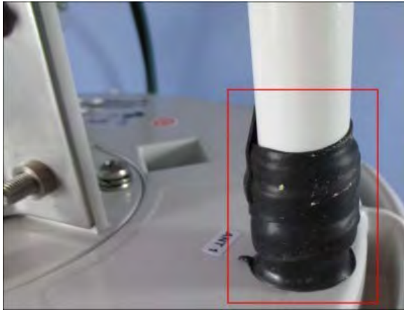
Figure 40: Layer of rubber insulation on antenna connection
