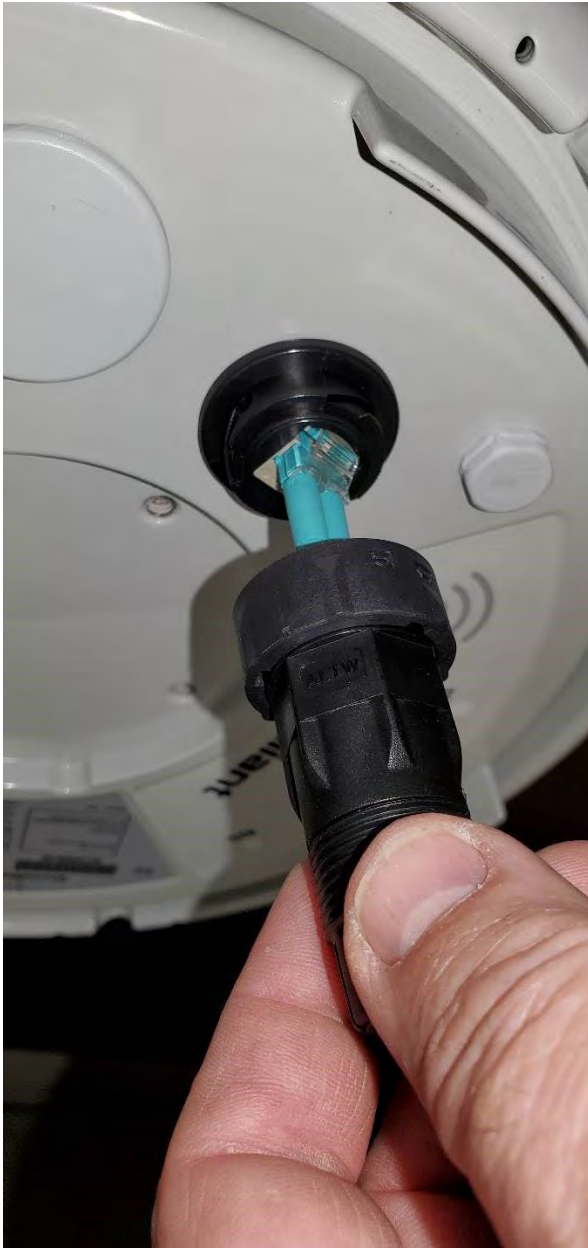
Figure 27: Connecting the Fiber Optic Cable to the female connector.
