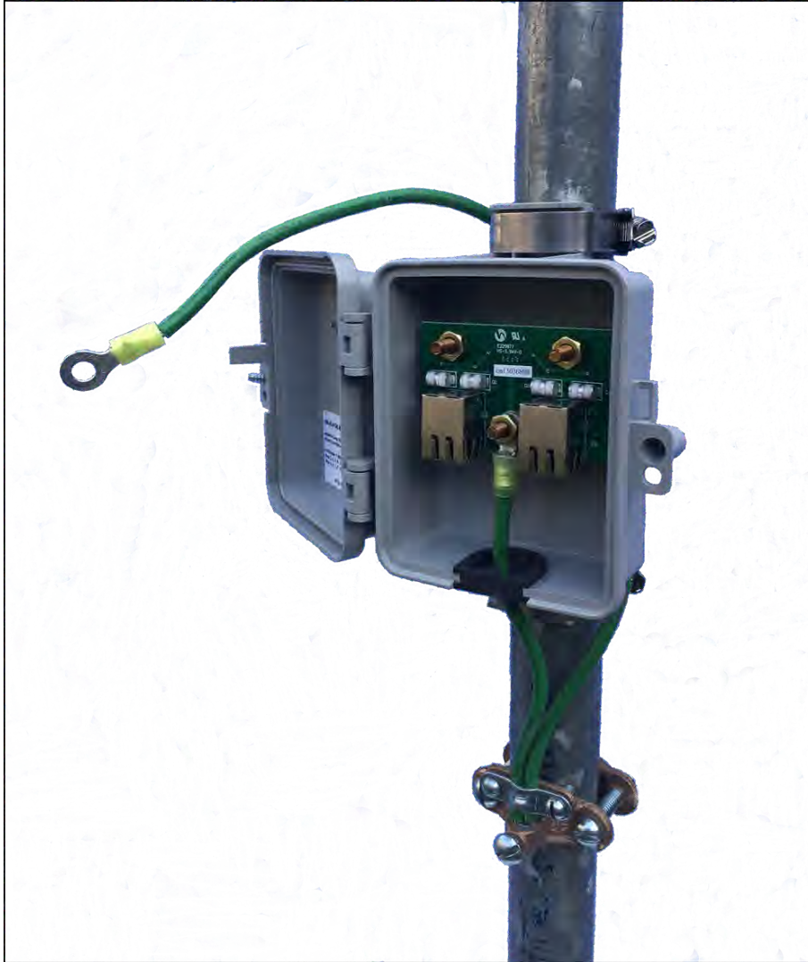
Figure 17: Attach the ground wire
