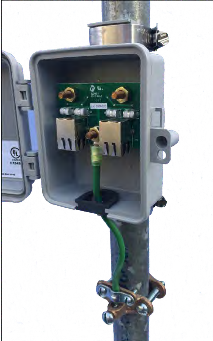
Figure 16: Assembled surge suppressor
