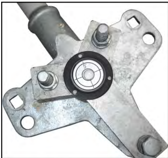
Figure 24: Magnetic level on adjustable leveling bracket
