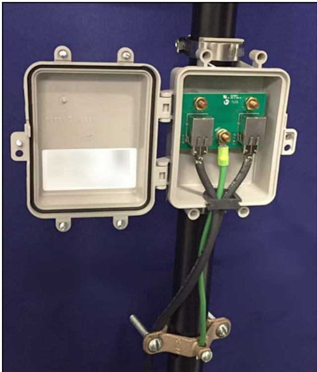
Figure 9: Citel Surge Suppressor with Gasket and Cables
