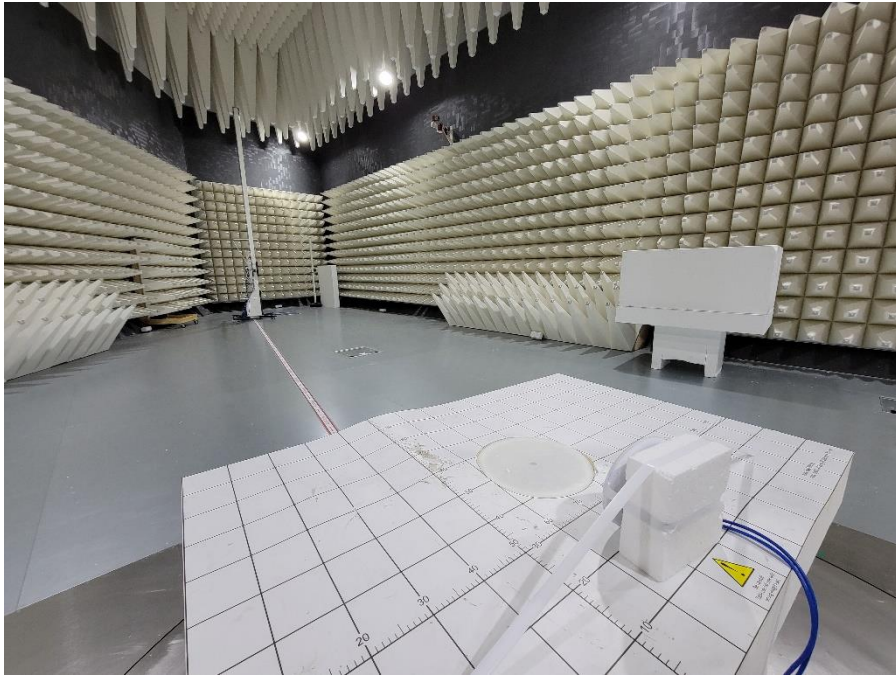
Photograph 1: View Test Set Up Radiated Emissions 30 – 1000 MHz
