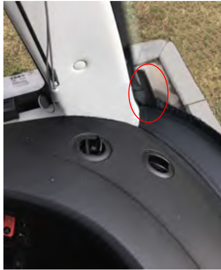
Figure 2-17 Inside installation of Mobile Network Antenna
