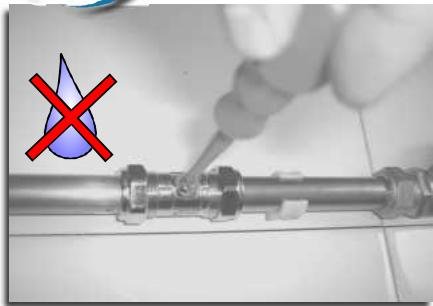
Locate your internal stop cock and close the water supply, check that all water using devices are turned off including hot water boilers and heating systems
