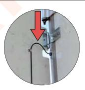
Proper Wiring Slack
