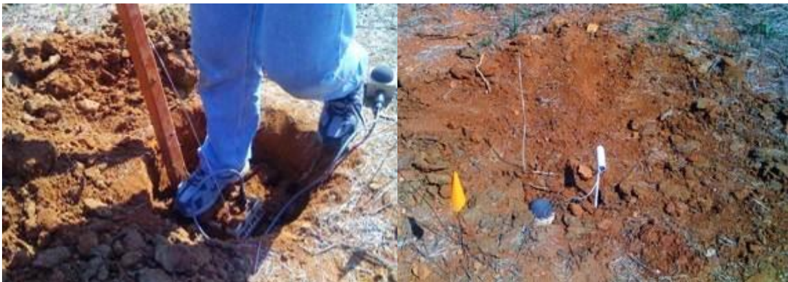
Figure 10 - Tightly pack soil around node during burial procedures
