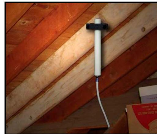
**Figure 5 - Mounting Signal Antenna to a Main Beam**
