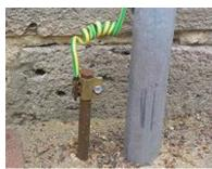
The mechanical installation must ensure that the Array is grounded to earth ground to dissipate static electric charge that may develop due to wind. In Step 3, you secured a grounding wire to the Array (see Step 3 if this has not been done).
