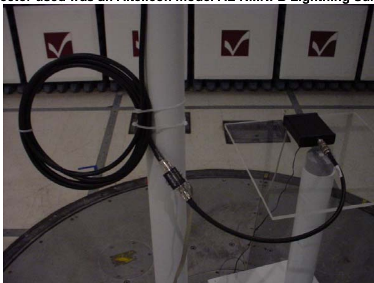
Close-up view of extra cable bundle and the surge protector installation. Surge protector used was an Altelicon model AL-NMNFB Lightning Surge Arrester.
