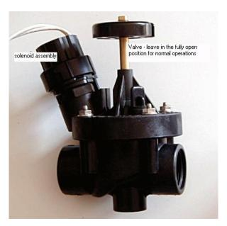
If the solenoid fails, you can still use it as a manual valve. Release the locking clip on the solenoid by lifting up on it. Unscrew the solenoid by turning it one half turn only, in a counter clockwise direction. This will allow water to flow. You can use the knob to regulate the flow or shut off flow.
