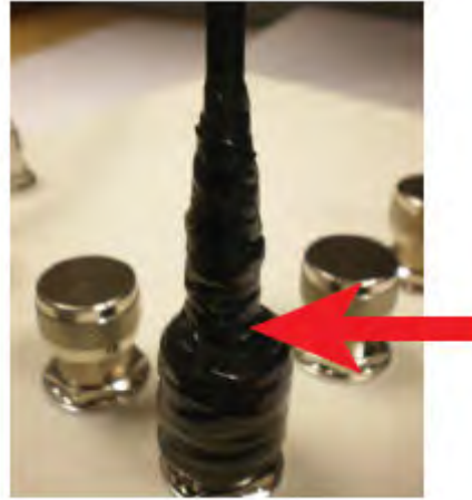
FIGURE 19 Wrapping the Electrical Tape
