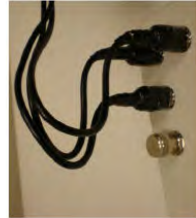
FIGURE 21 Creating Cable Drip Loops
