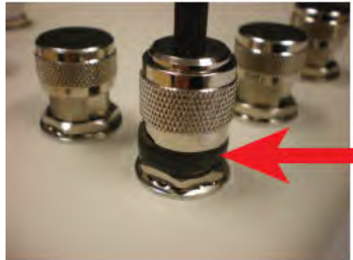
FIGURE 13 Wrapping the Exposed Connector Threads
