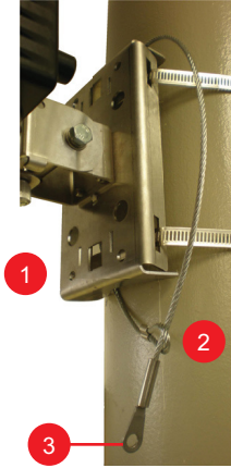
Figure 28. Secured safety cable
