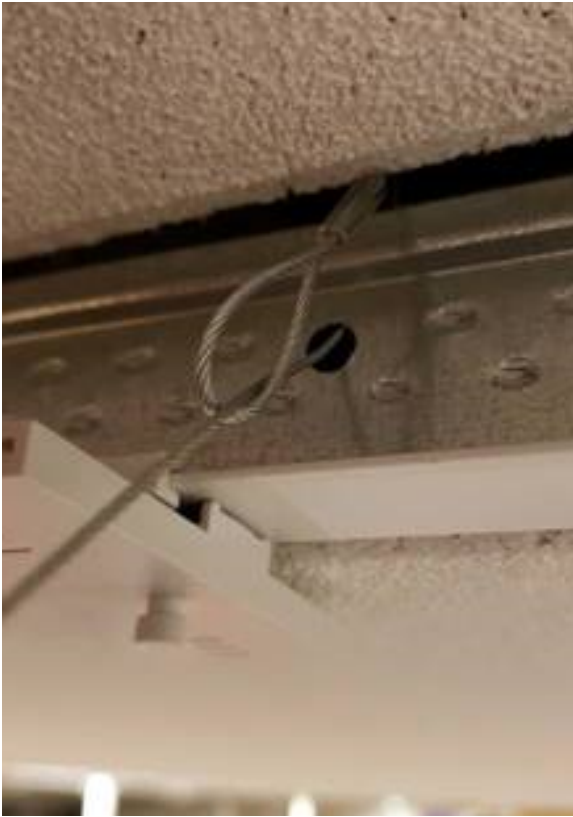
FIGURE 3 Attaching the Cable to a Structurally Sound Anchor
