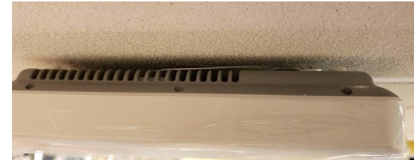
FIGURE 6 Tucking Excess Cable
