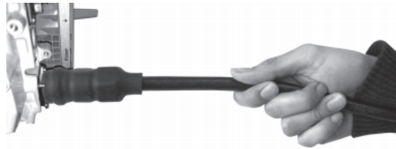
FIGURE 17 Fully Deployed Cold Shrink
