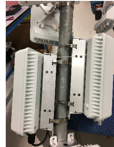
FIGURE 10 Attaching APs to the Pole
