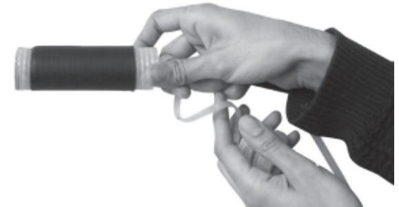
FIGURE 14 Evening the Plastic Tab with the Shrink Sleeve
