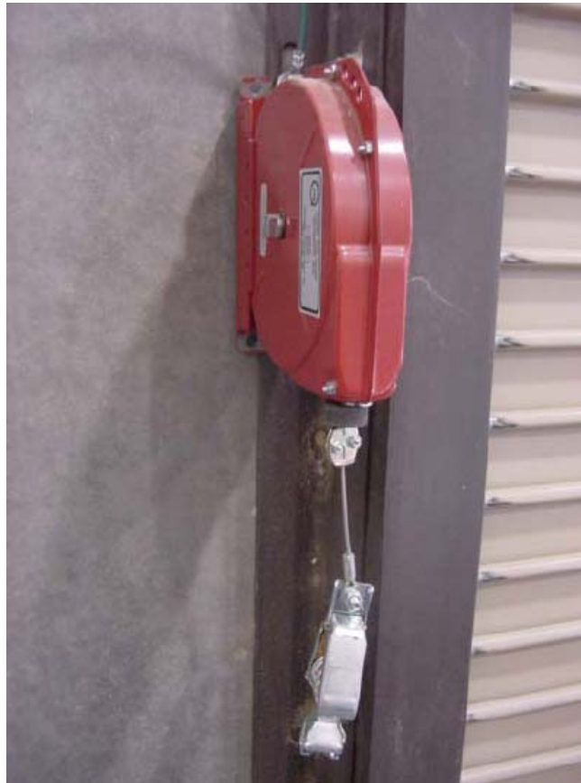
Figure 3.1 – Ground Wire clip
