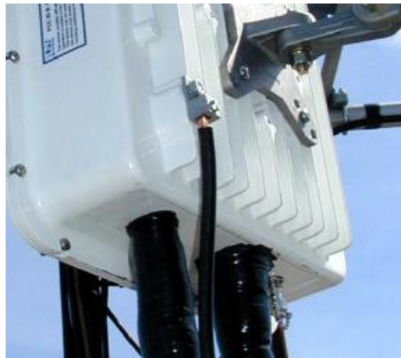
Figure 5-10 ODU Ground Lug
