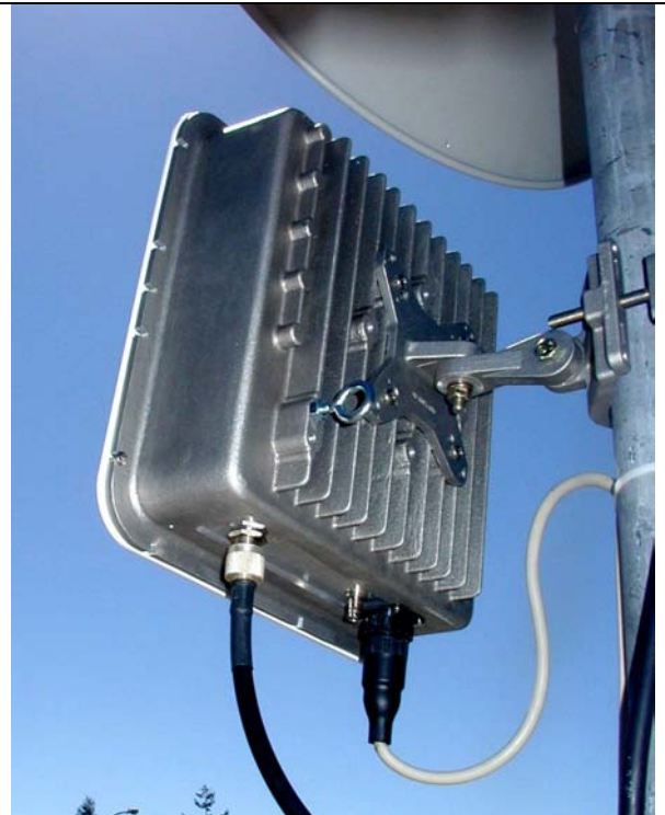
Figure 4-5 Typical ODU Mast Mount Mechanical Installation
