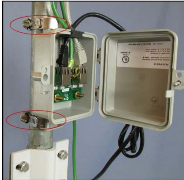
Figure 8 Hose clamps to mount Citel surge suppressor
