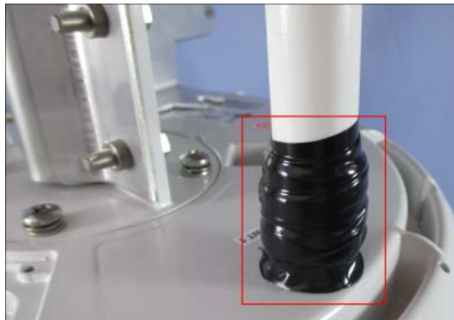
Figure 29 Outer layer of tape on antenna connection
