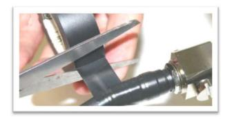
**Note:** To make a watertight connection, keep tension in the butyl mastic when you stretch it over the cable and connector.
