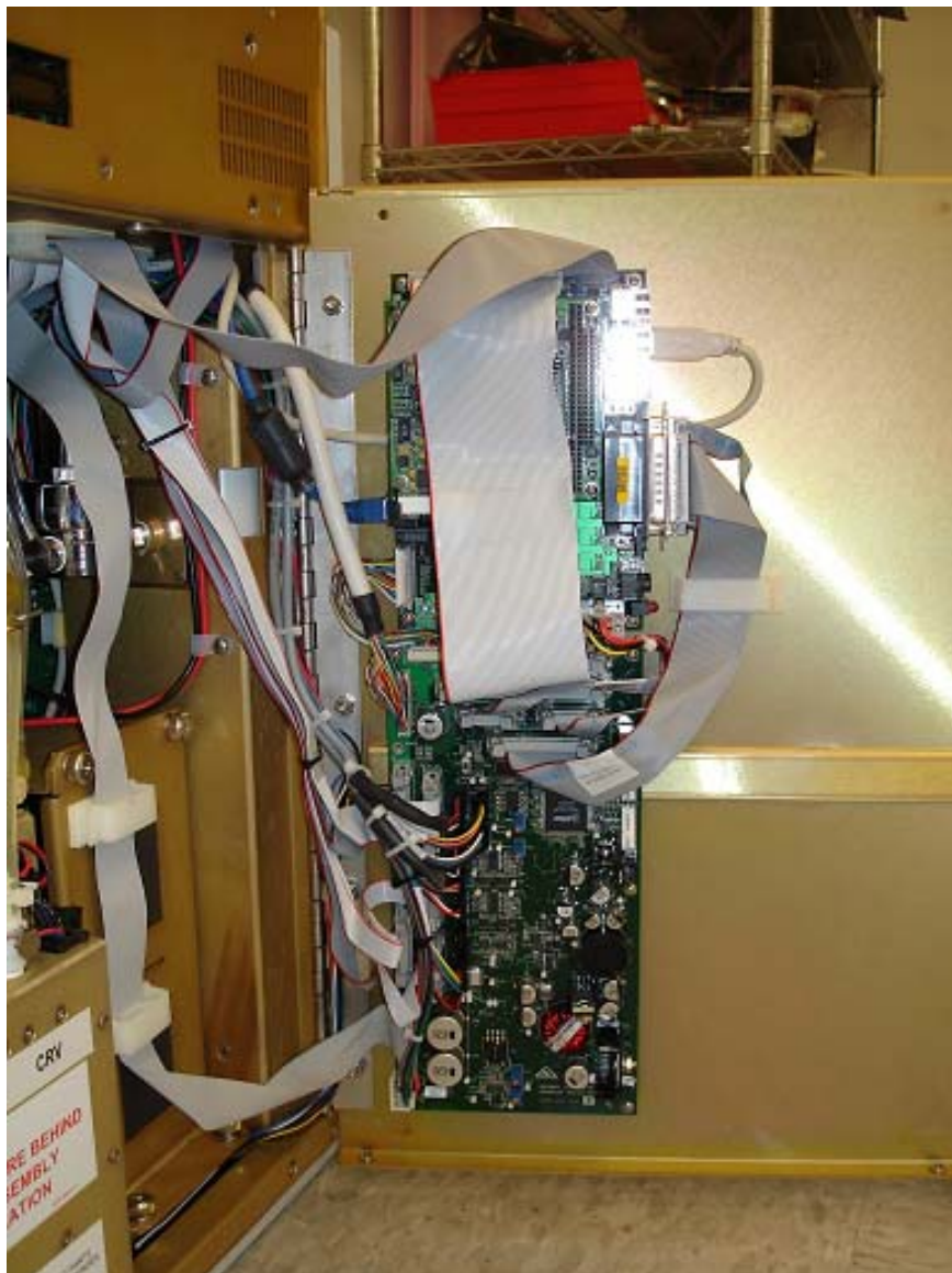
0036-0010 Recover BP – Inside Door View (Close)
