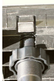
Figure 2.27 Threading the mounting nut
