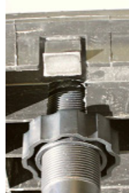
Figure 2.4 Threading the antenna nut
