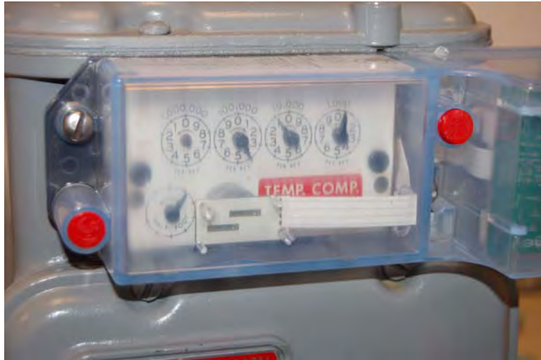
Figure 6 - 24. Meter module with tamper seals installed
