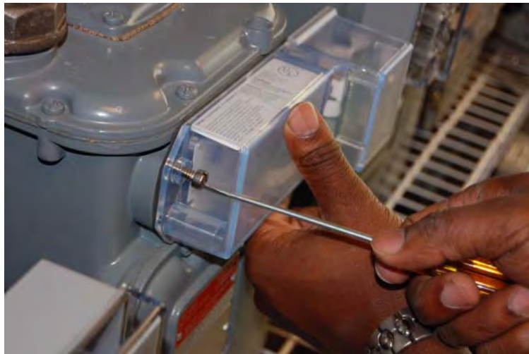
Figure 6 - 21. Installing the first Gas LX Cover mounting screw
