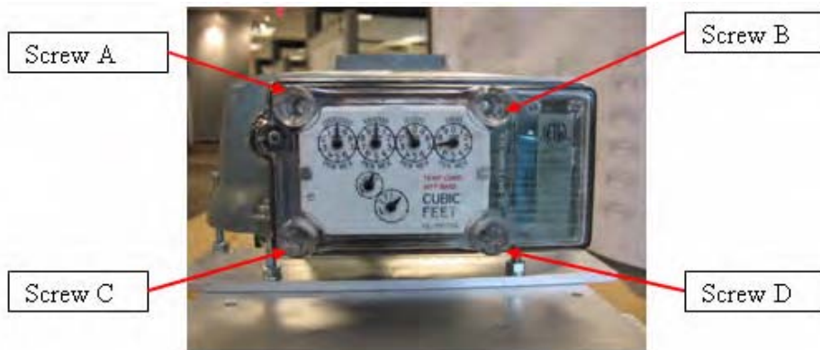
Figure 5.23 Rockwell/Equimeter/Sensus: two-screw configuration
