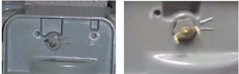
Figure 5.45 Lancaster/National: Installation of New Coupler
