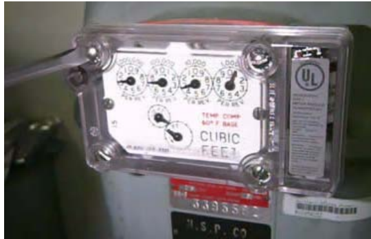
Figure 5.22 Rockwell/Equimeter/Sensus: Installing the Meter Module cover
