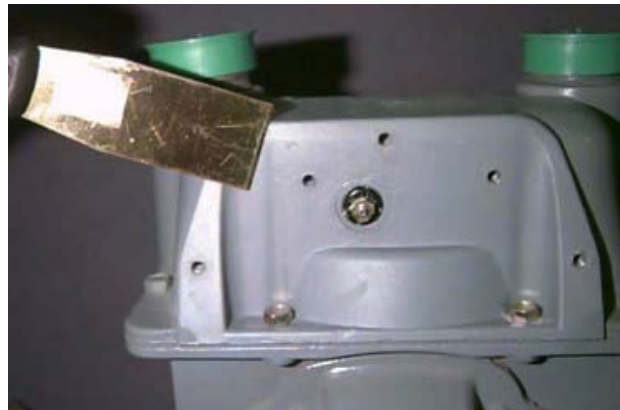
Figure 5.44 Lancaster/National: Removal of index cover gasket
