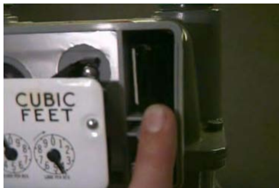
Figure 5.36 Sprague/Schlumberger/Actaris: Battery Correctly Installed
