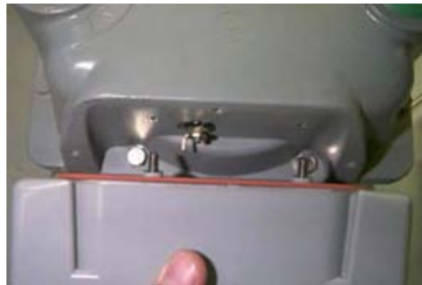
Figure 5.31 Sprague/Schlumberger/Actaris: Alignment of the meter drive dog and screws
