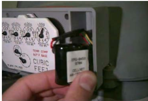
Figure 5.20 Rockwell/Equimeter/Sensus: Correct battery orientation (connector on top)
