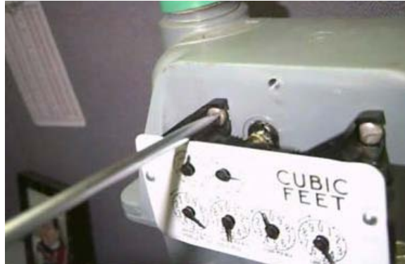
Figure 5.28 Sprague/Schlumberger/Actaris: Removing the index
