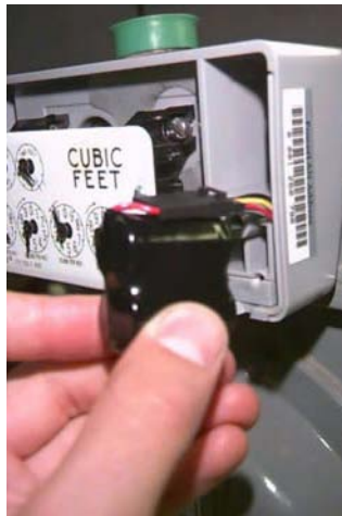
Figure 5.35 Sprague/Schlumberger/Actaris: Correct Battery Orientation
