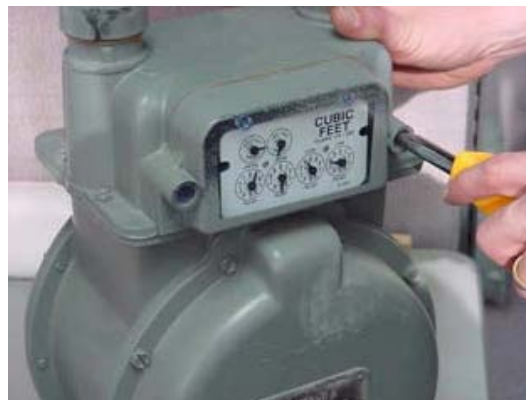
Figure 5.42 Lancaster/National: Removing the index cover
