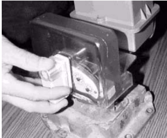
Figure 6.18 Rockwell/Equimeter/Sensus: meter module installing Index cover
