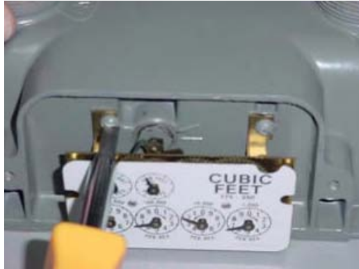
Figure 5.43 Lancaster/National: Removing the index
