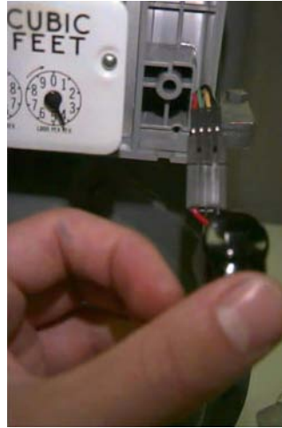
Figure 5.49 Lancaster/National: Connecting the Battery
