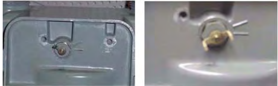
Figure 5.45 Lancaster/National: Installation of New Coupler
