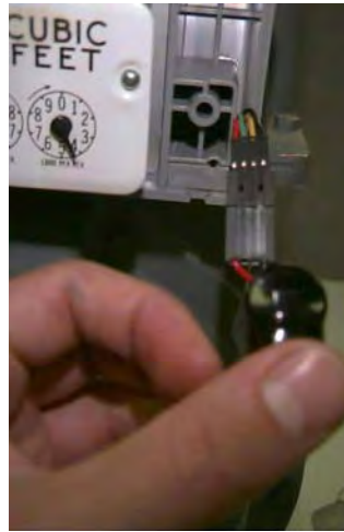
Figure 5.34 Sprague/Schlumberger/Actaris: Connecting the Battery
