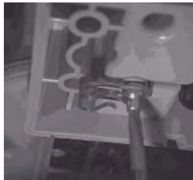
Figure 5.6 American: Attaching the Meter Module onto the meter by screwing in two stand-off fasteners
