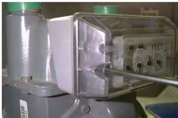
Figure 5.52 Lancaster/National: Fasten Cover Screws and Insert Tamper seals
