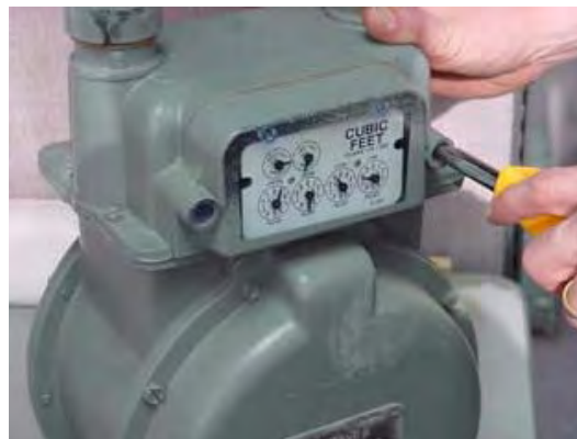
Figure 5.42 Lancaster/National: Removing the index cover
