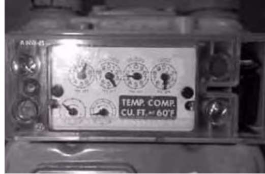
Figure 5.12 American: Meter module with cover and tamper seals installed
