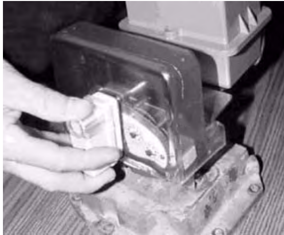
Figure 6.18 Rockwell/Equimeter/Sensus: meter module installing Index cover
