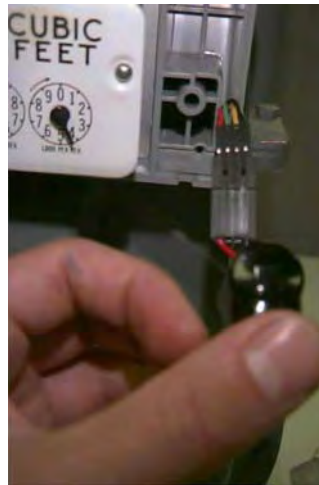
Figure 5.49 Lancaster/National: Connecting the Battery
