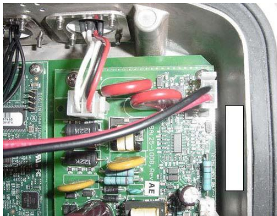
Figure 5 - 3. RF Filter retrofit remove gasket and battery cables
