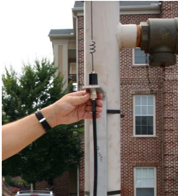
Figure 4 - 10. Attaching RF cable
