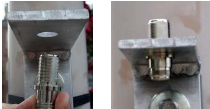
Figure 4 - 6. Attaching bulkhead connector
