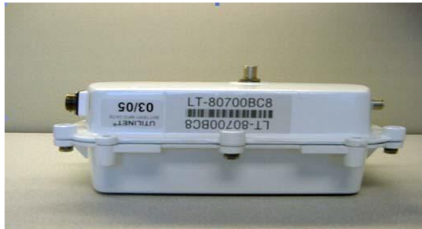
Figure 5 - 11. New battery date label affixed to concentrator enclosure
