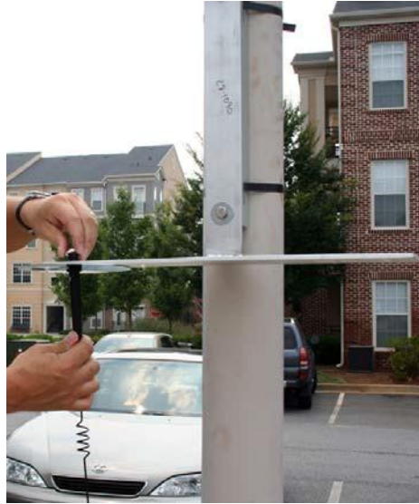
Figure 4 - 9. Connecting a LAN antenna
