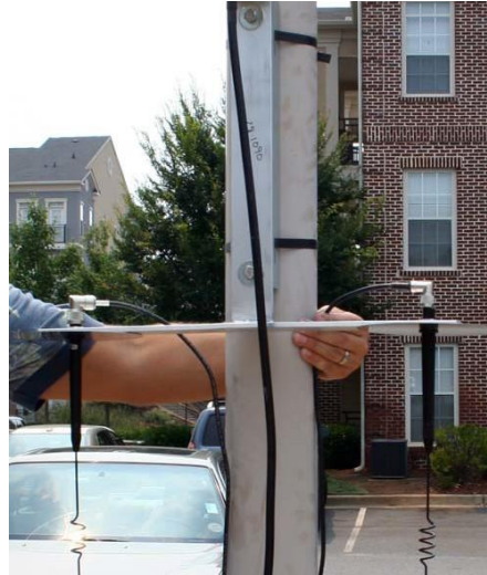
Figure 4 - 11. Attaching right-angle end of cable
