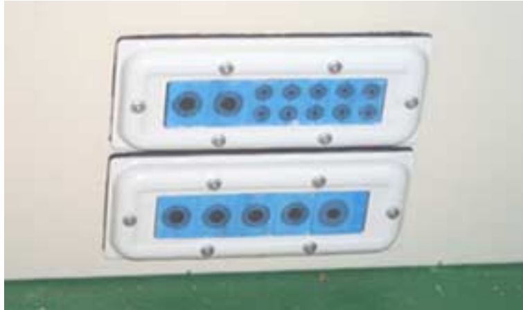
Figure 4-5: Roxtec Assembly
