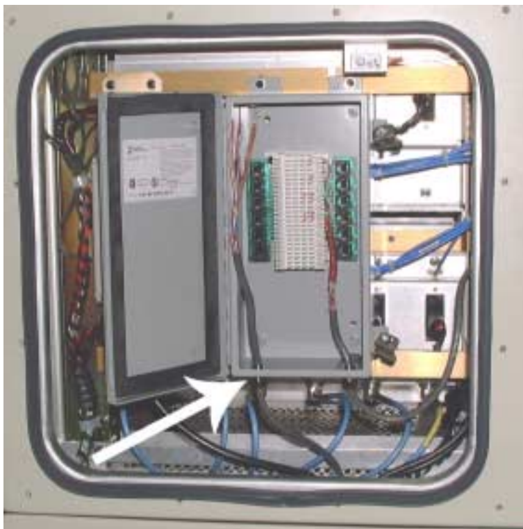
Figure 5-4: T1 Termination Box Open
