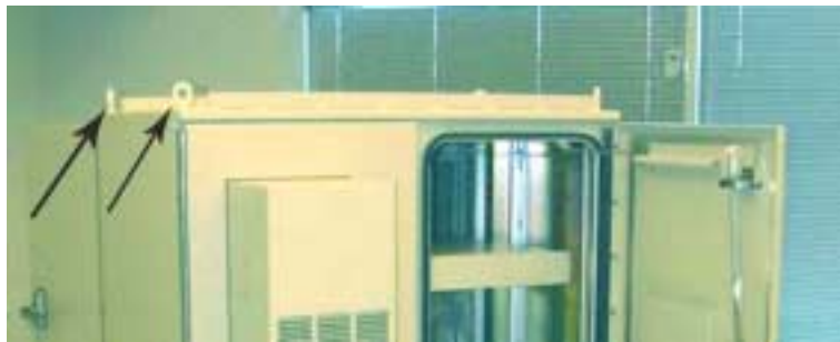
Figure 3-5: Eyebolts for Lifting Cabinet
