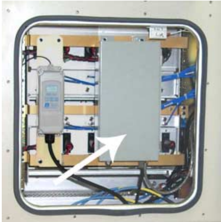
Figure 5-3: T1 Termination Box — Rear View
