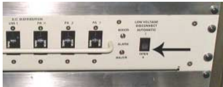
Figure 7-7: Low Voltage Disconnect
