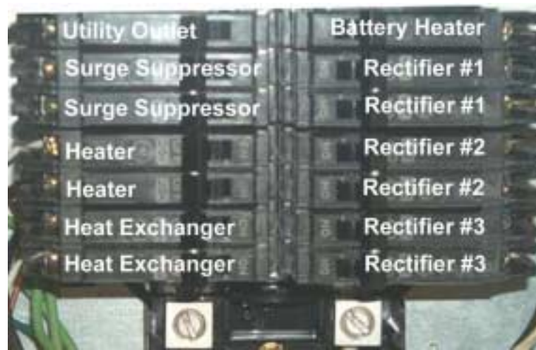
Figure 7-6: Turning AC Breakers On
