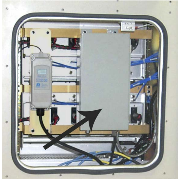
Figure 5.3 T1 Termination Box — Rear View
