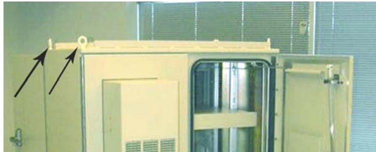
Figure 3.5 Eyebolts for Lifting Cabinet
