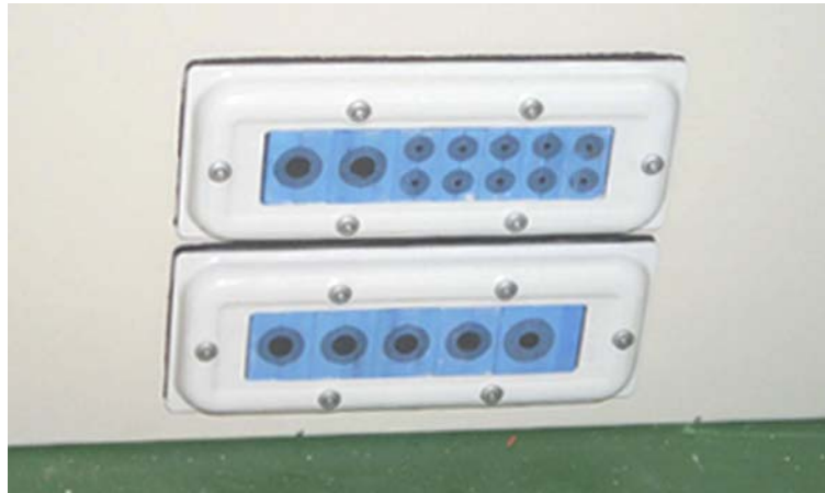
Figure 4.5 Roxtec Assembly
