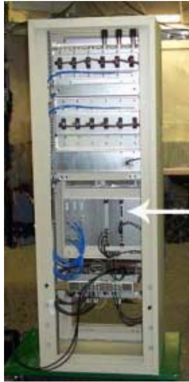
Figure 6-1: Cabinet with Alarm Connector — Rear View
