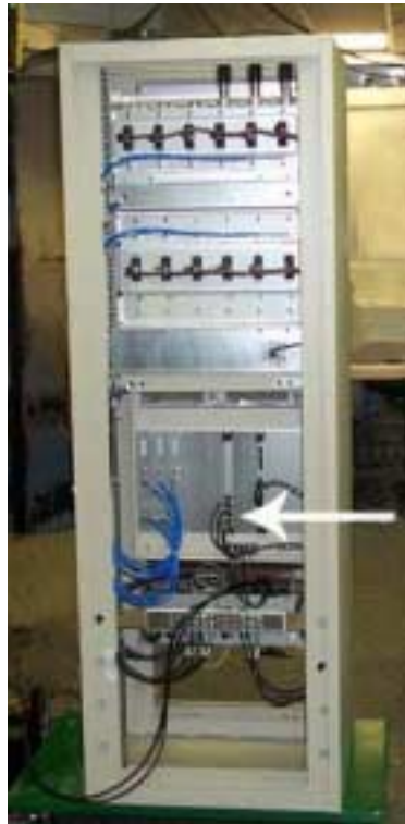
Figure 5-1: Cabinet with T1 Connectors — Rear View
