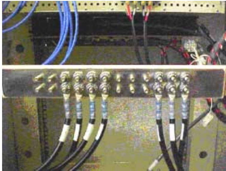
Figure 4-14: Ground Bus Bar
