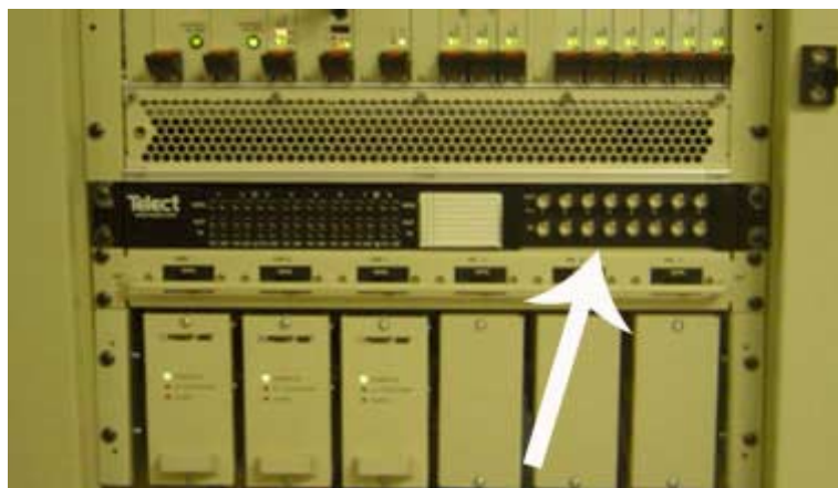
Figure 5-4: Backhaul Access Panel — Front View
