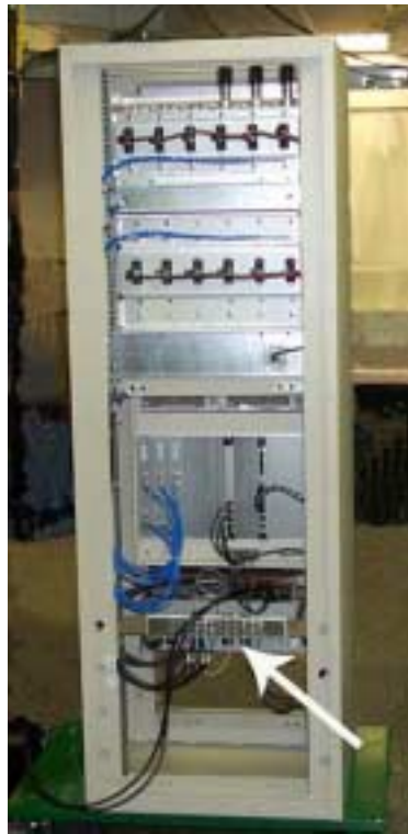
Figure 4-13: Cabinet with Ground Bus Bar — Rear View
