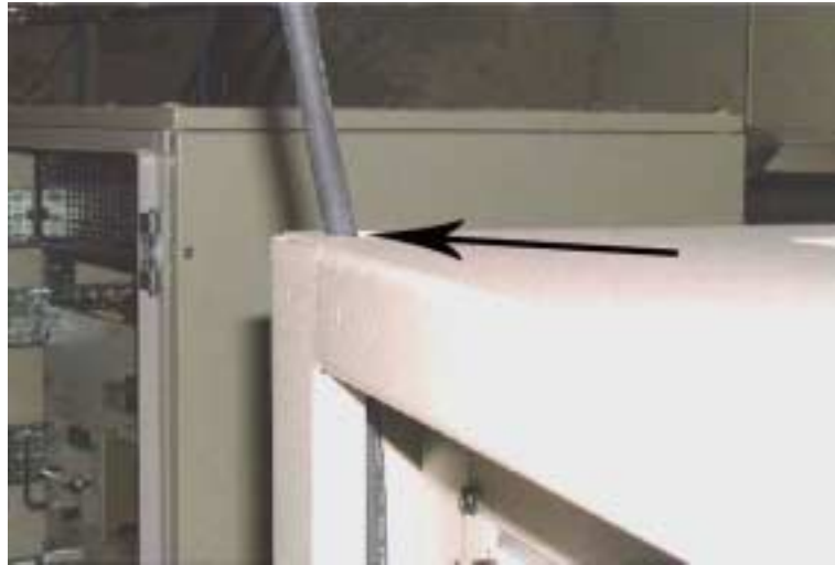
Figure 4-1: Cable Entry Port
