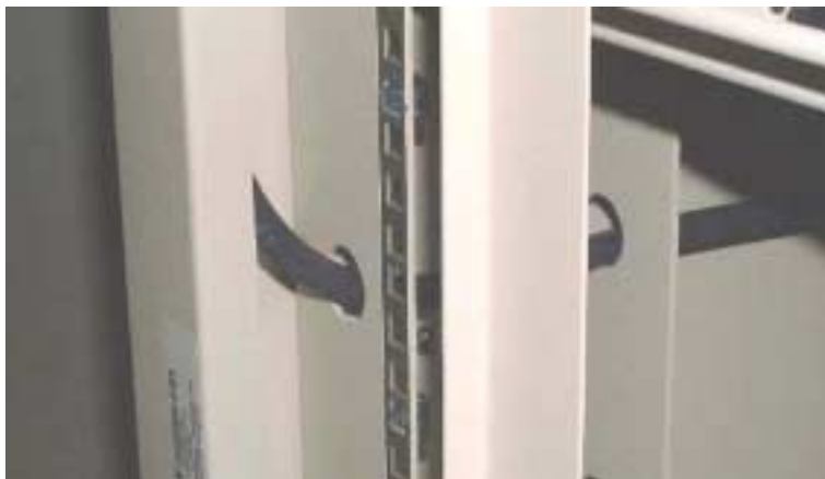
Figure 4-4: Cable Routed Through Structure
