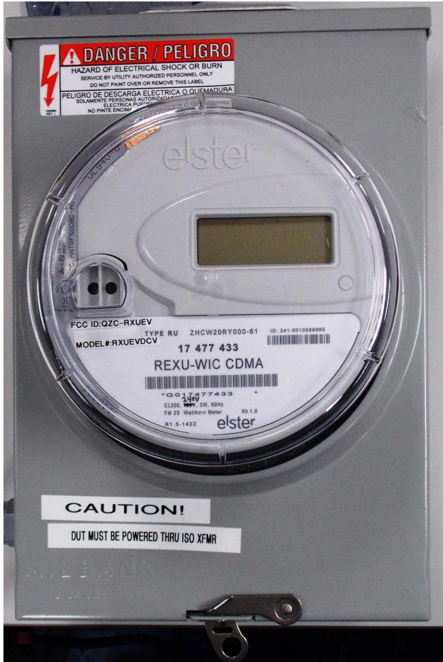
REXUniversal ® installed in typical enclosure
