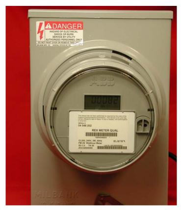
Figure 1 – Picture of a REX meter in an electrical socket
