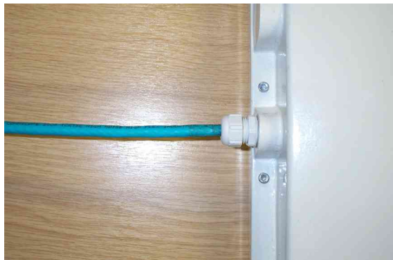
Step 4: Screw on the clamping nut and tighten to ?? Nm
