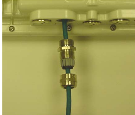
Step 2: Insert the RJ45 connector making sure that the locking tab snaps home
