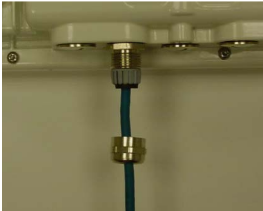
Step 3: Screw in the body of the weather proofing gland and tighten
