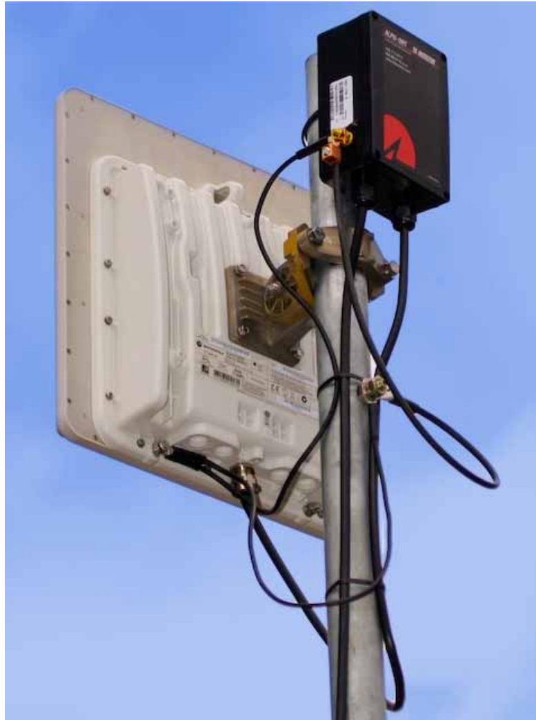
Figure 79 - Upper Grounding Configuration
