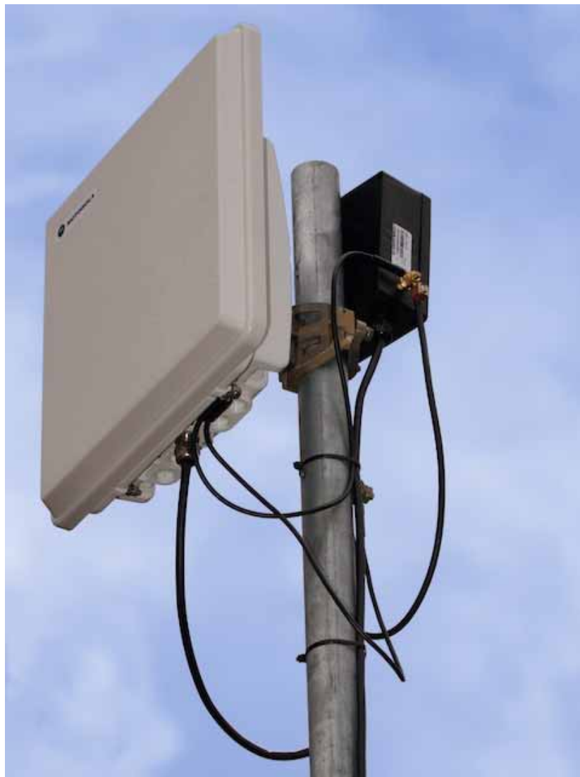
Figure 2 - PTP 400 Series Bridge Outdoor Unit (ODU)
