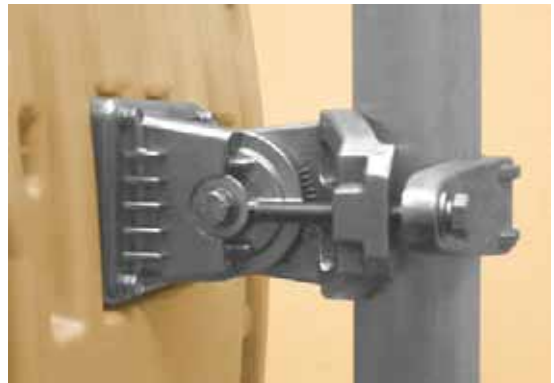
Step 2: Mate the unit to the bracket and tighten the nut and bolt.
