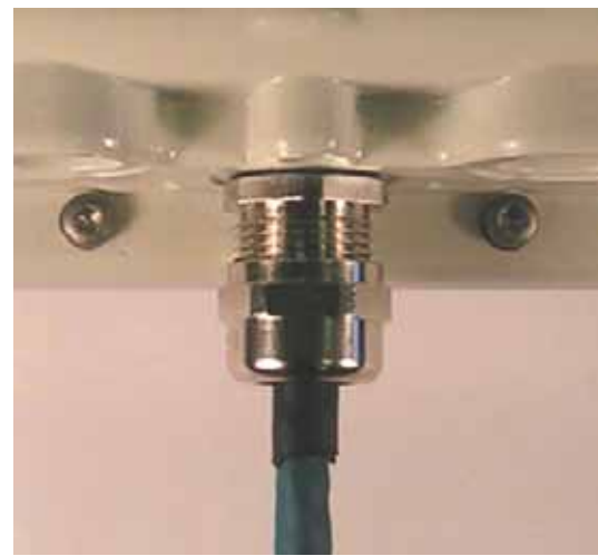
Step 4: Screw on the clamping nut and tighten
