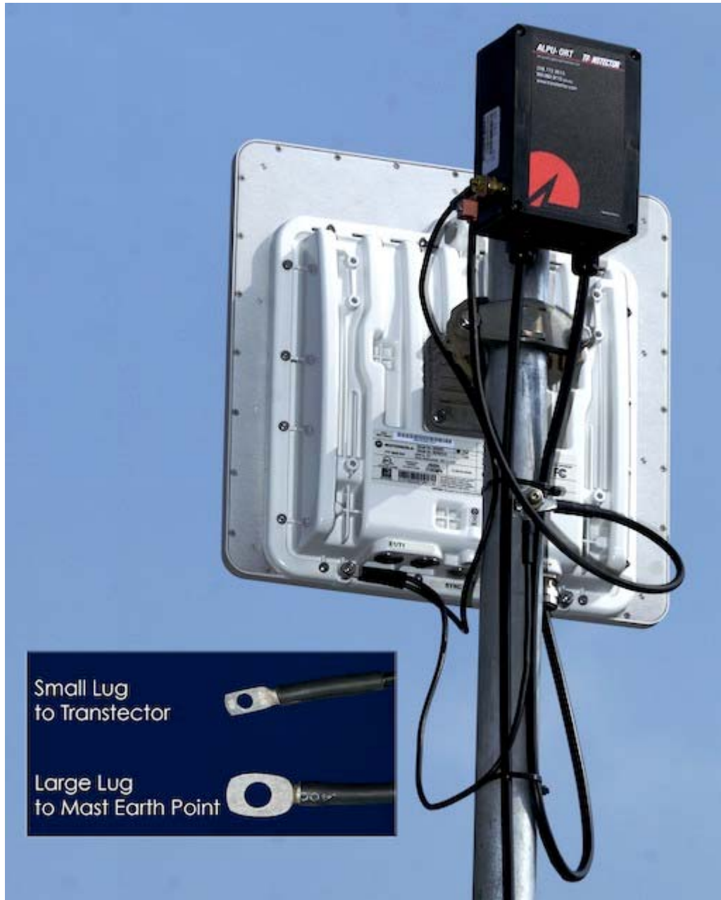
Figure 96 - Upper Grounding Configuration
