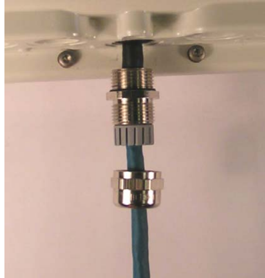
Step 2: Insert the RJ45 connector making sure that the locking tab snaps home
