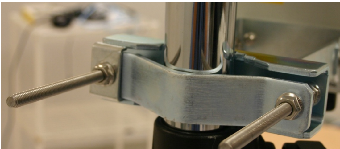
Figure 103 Attaching the AP antenna lower bracket to the pole
