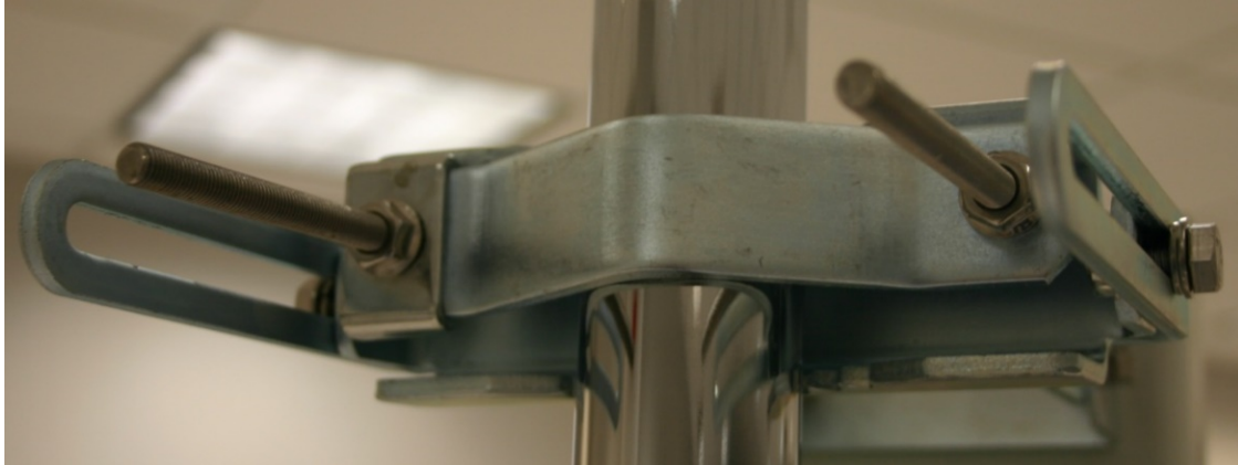
Figure 102 Attaching the AP antenna upper bracket to the pole
