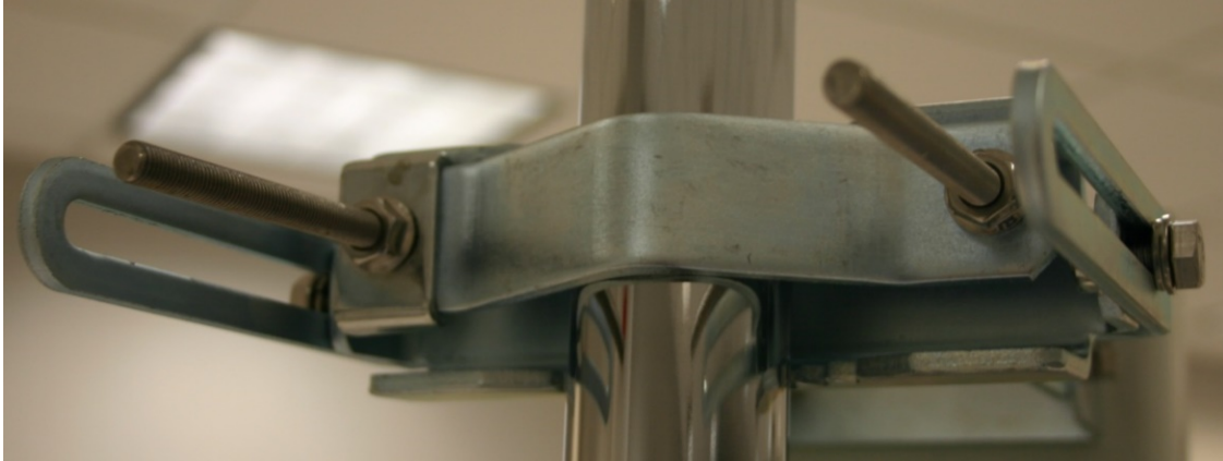
Figure 74 Attaching the AP antenna upper bracket to the pole
