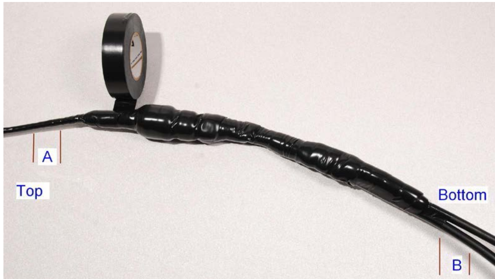
Figure 114 Wrapping PVC tape around the GPS adapter cable joint
