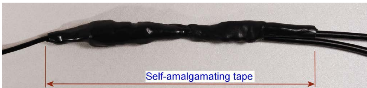
Figure 113 Wrapping self-amalgamating tape around the GPS adapter cable joint
