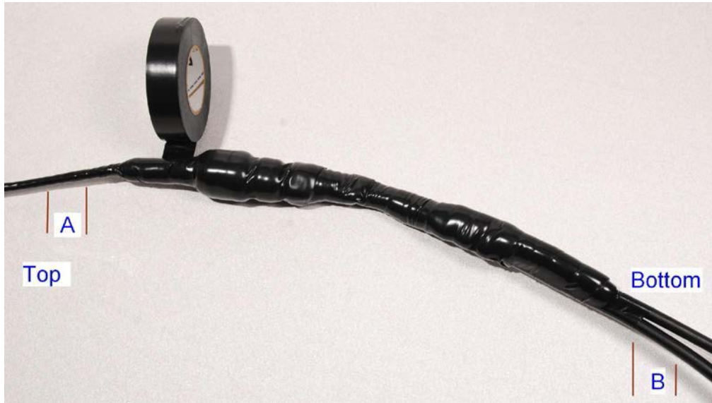
Figure 117 Wrapping PVC tape around the GPS adapter cable joint
