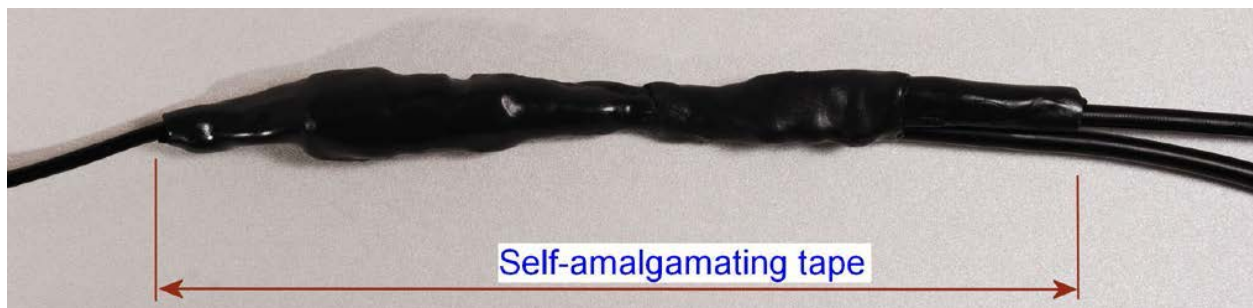
Figure 116 Wrapping self-amalgamating tape around the GPS adapter cable joint
